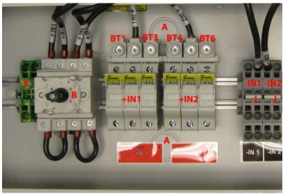
Figure 2.06a - DC Array Connection PVI-10.0-I-OUTD-S1-US/CAN-XXX-YY
