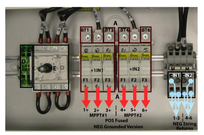
Figure 3.06 - DC Array Connection PVI-10/12-I-OUTD-S2-US/CAN--XXX using Fuses
