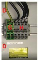
Figure 2.04 - Switchbox Wiring Connection Details PVI-10.0-I-OUTD-S1-US/CAN-XXX-YY
