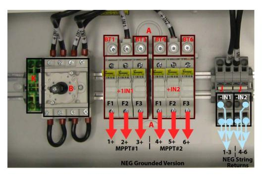
Figure 2.06b- DC Array Connection *PVI-10.0-I-OUTD-S1-US/CAN-XXX-YY*
