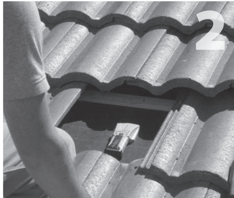
2 Locate and mark center of rafter.
