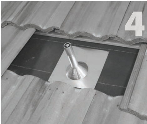
Install the sub-flashing over the post, making sure the edge closest to the cone is on the downhill side.
