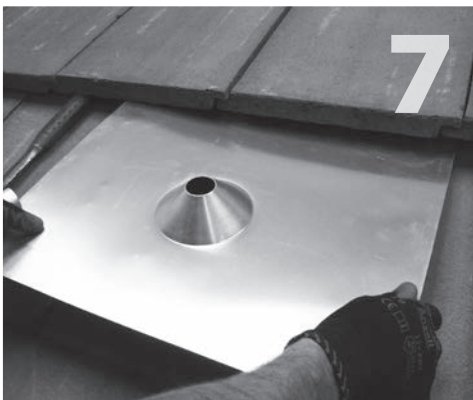
7 Cut a hole in the removed tile, with room to get the post through. Place cut tile back in position. Insert post and tighten into place. Install the 18"x 18" flashing and apply sealant around the opening.
