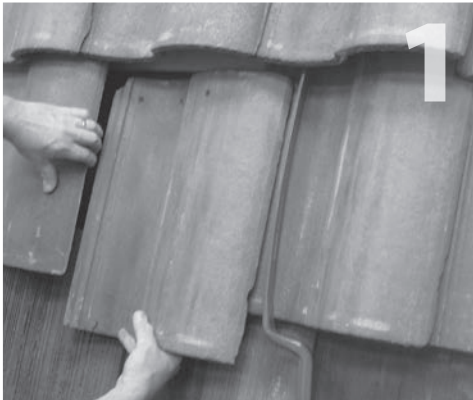
1 Remove tile at selected location of mount.
