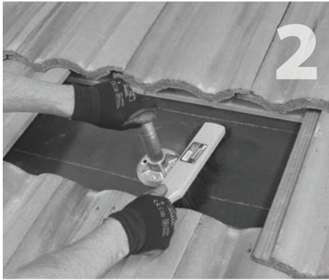
Clean away dust and debris around QBBase.
