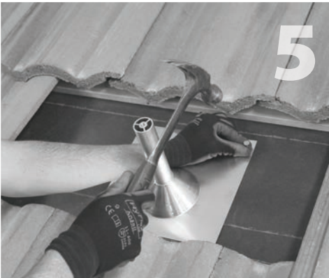
Fasten the sub-flashing into place with two roofing nails, one in each top corner.
